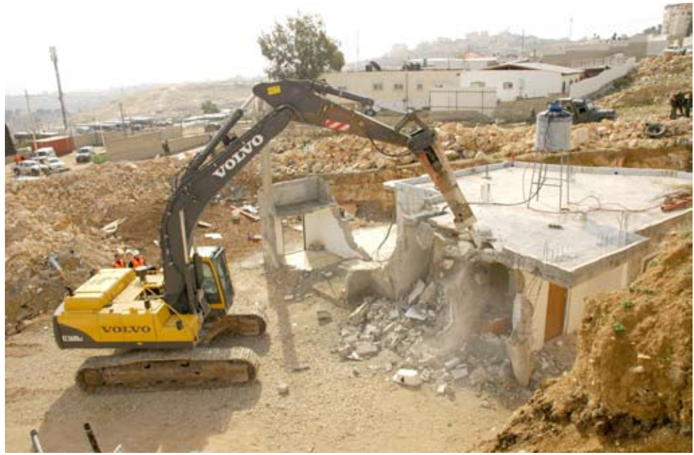
House demolition in Jerusalem, 2010 (© ICHAD)
