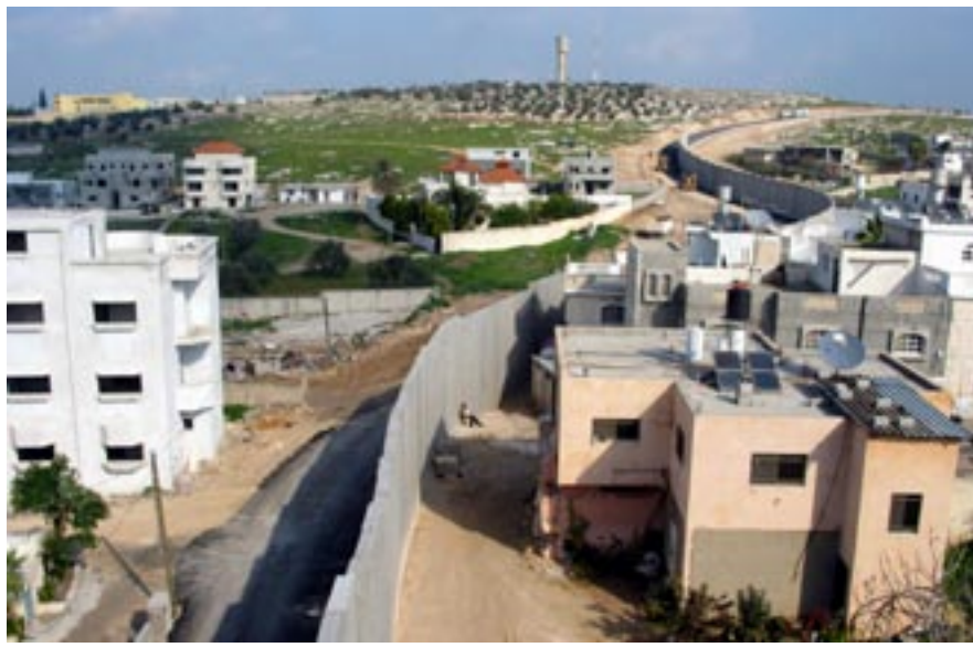
The Wall running through Palestinian houses in the West Bank. © al-Ayyam
