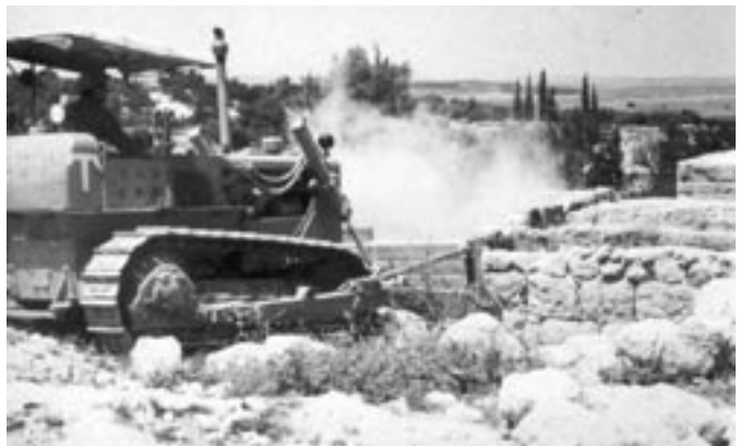
Israeli bulldozers level the village of Imwas in 1967. © www.palestineremembered.com.
