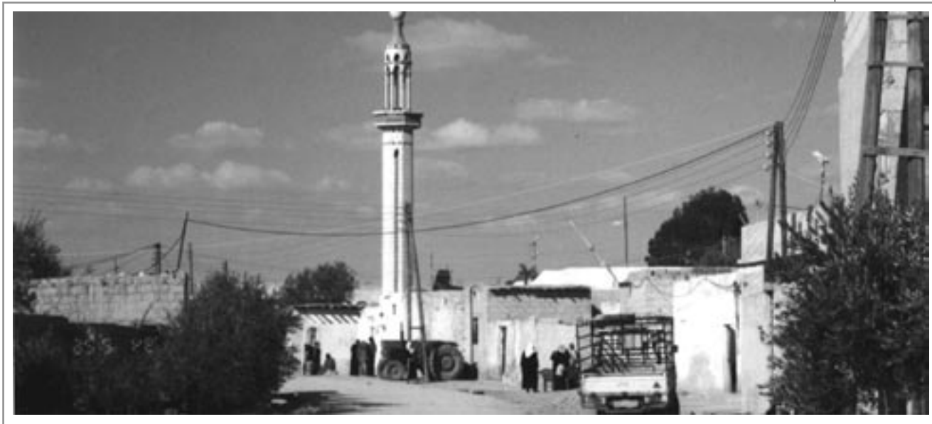
Housing in Ein al-Tal, Aleppo, Syria, for refugees from Neirab camp which is being rehabilitated due to poor housing standards. © Ron Wilkinson.
